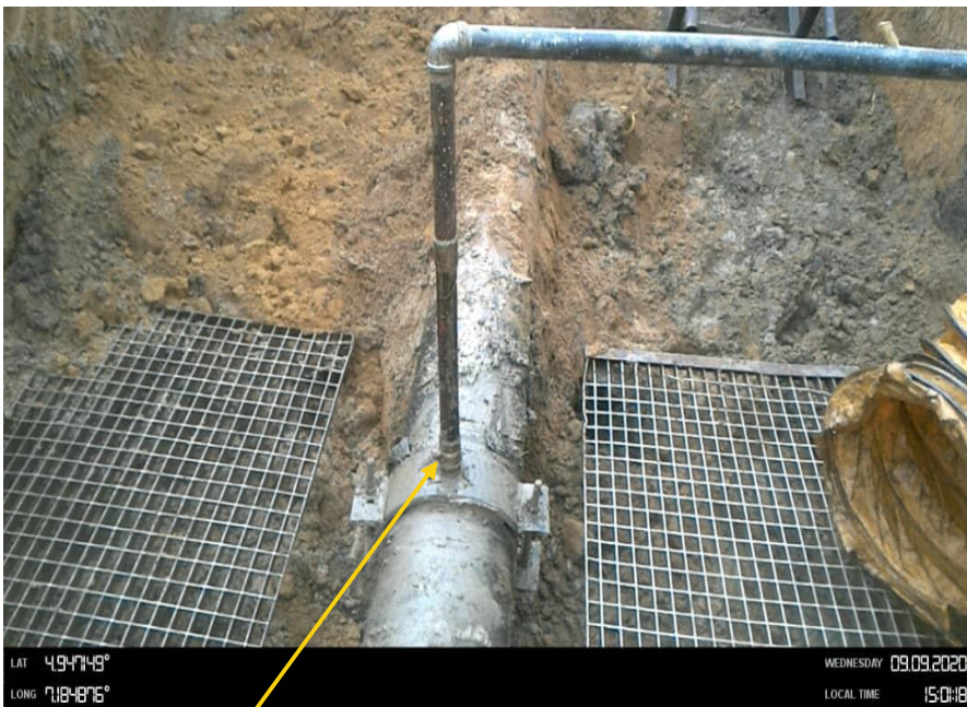
Close-up: Crude oil theft point installed at 12 o'clock position on 12" Imo River2 - Ogale Pipeline at Umuololo. Picture was taken during Joint Investigation on 9th September 2020.
