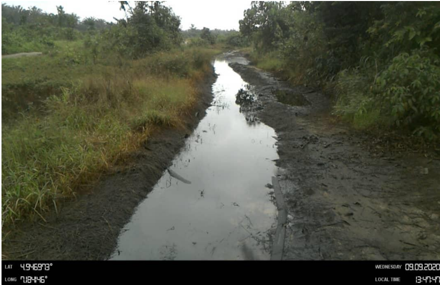
Overview: Part of spill impact on 12" Imo River2 - Ogale Pipeline at Umuololo. Picture was taken during Joint Investigation on 9th September 2020.
