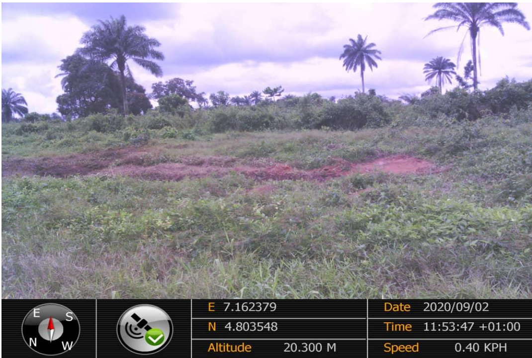
Overview: Part of spill impact on 24" Nkpoku - Bomu Pipeline at Agbeta. Picture was taken during Joint Investigation on 2nd September 2020.
