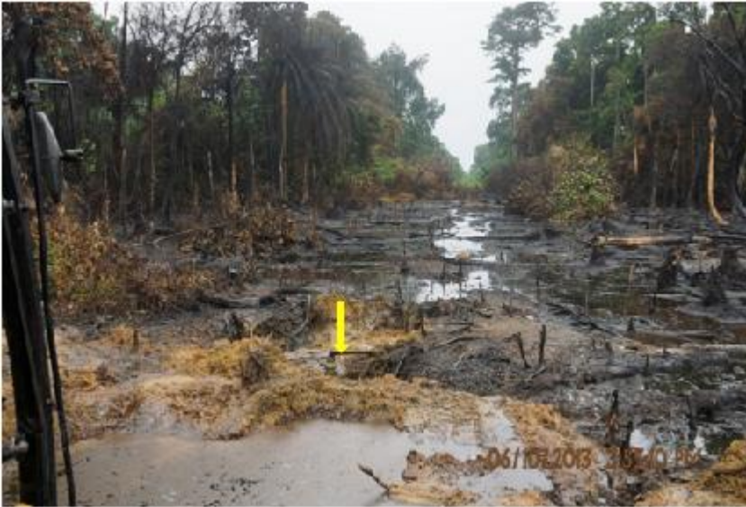
Overview: Part of spill point 1 impact on 20" Otumara Escravos Pipeline at Ajudaibo. Picture was taken during Joint Investigation of 6th October 2013.
