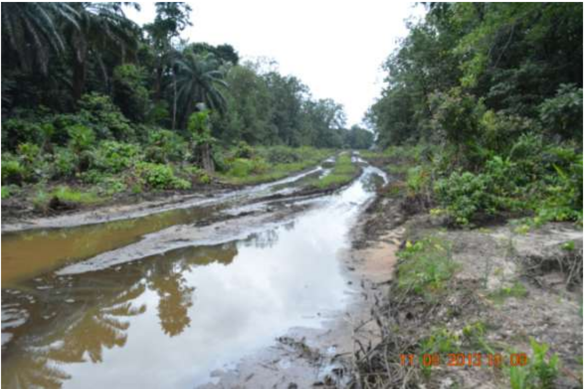
Overview: Part of spill impact on 20" Otumara-Escravos pipeline right of way at Ugborodo/Ugboegungun. Picture was taken during Joint Investigation of 11 th September 2013.
