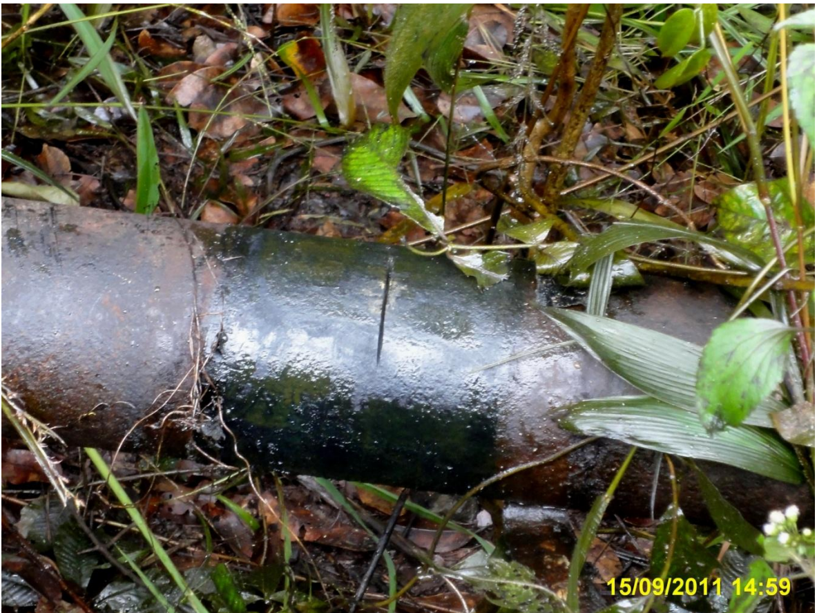
Overview: Initial hacksaw cut previously clamped on Adibawa Well 10S flowline at Edagberi. Picture was taken during Joint Investigation of 15th September, 2011.
