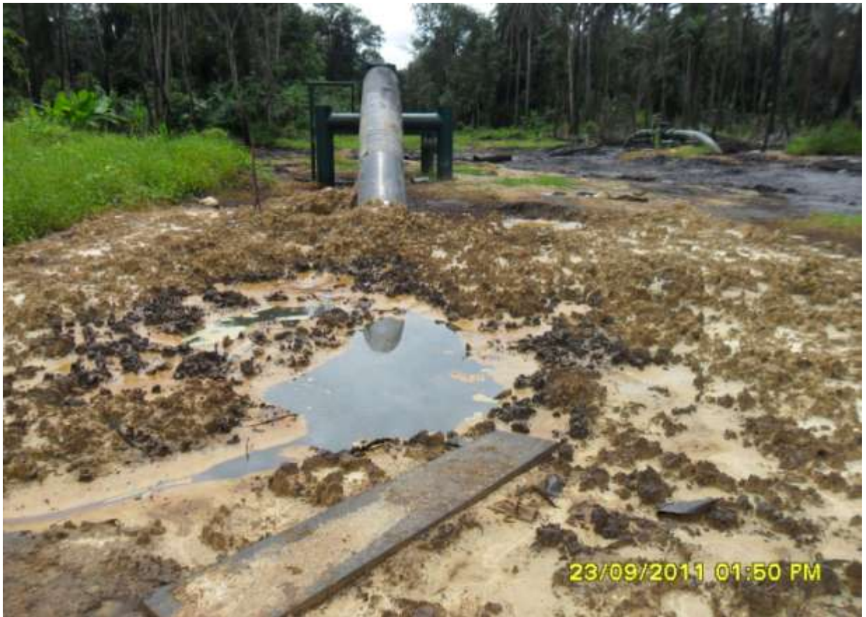
Overview: Part of spill incident impact at 20" Kolocreek–Rumuekpe Pipeline right of way at Ogbogolo. Picture was taken during JIV of 23 rd September, 2011
