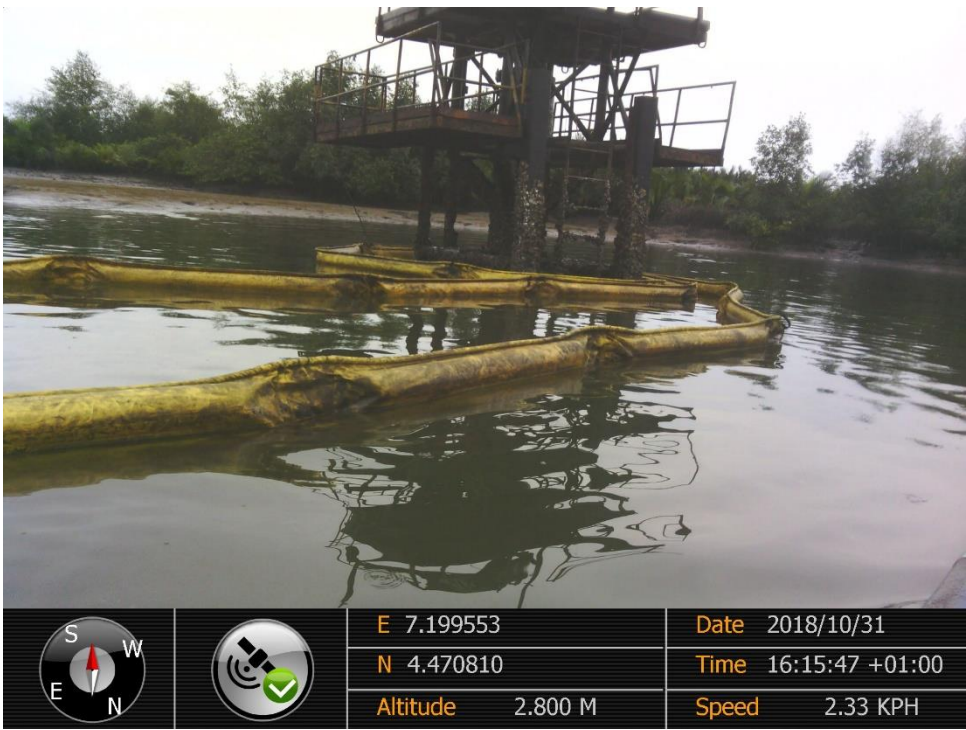
Overview: Part of spill impact on 4" Bonny Well 18S Flowline Riser at Oloma. Picture was taken during Joint Investigation of 31 st October 2018.
