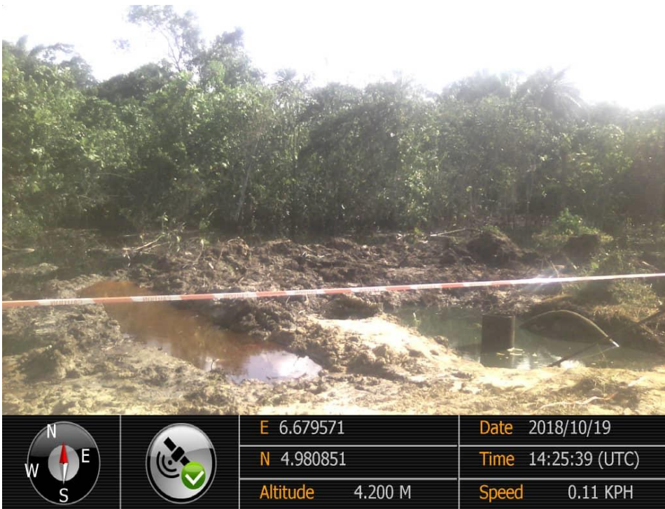
Overview: Part of spill impact on 20" Kolocreek-Rumuekpe Pipeline at Imogu-Rumuekpe. Picture was taken during Joint Investigation of 19 th October 2018.
