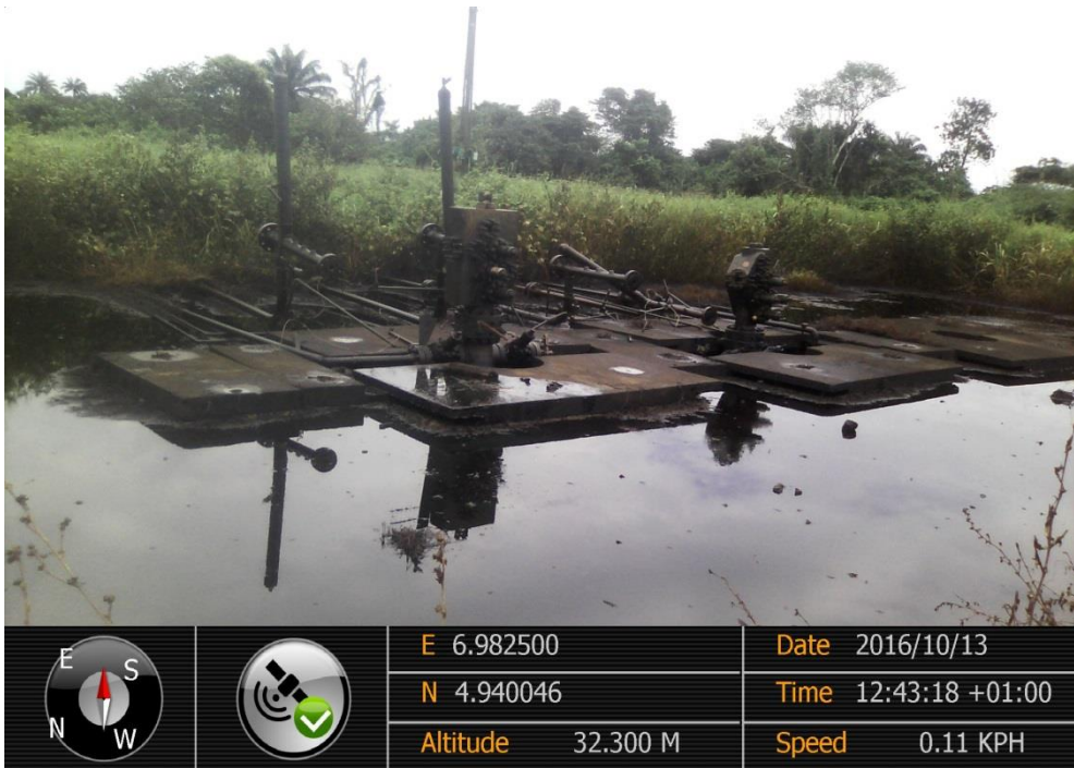
Overview: Part of spill impact on Agbada 1 Well 13 and 18 Wellheads at Omunike. Picture was taken during Joint Investigation of 13 th October 2016.
