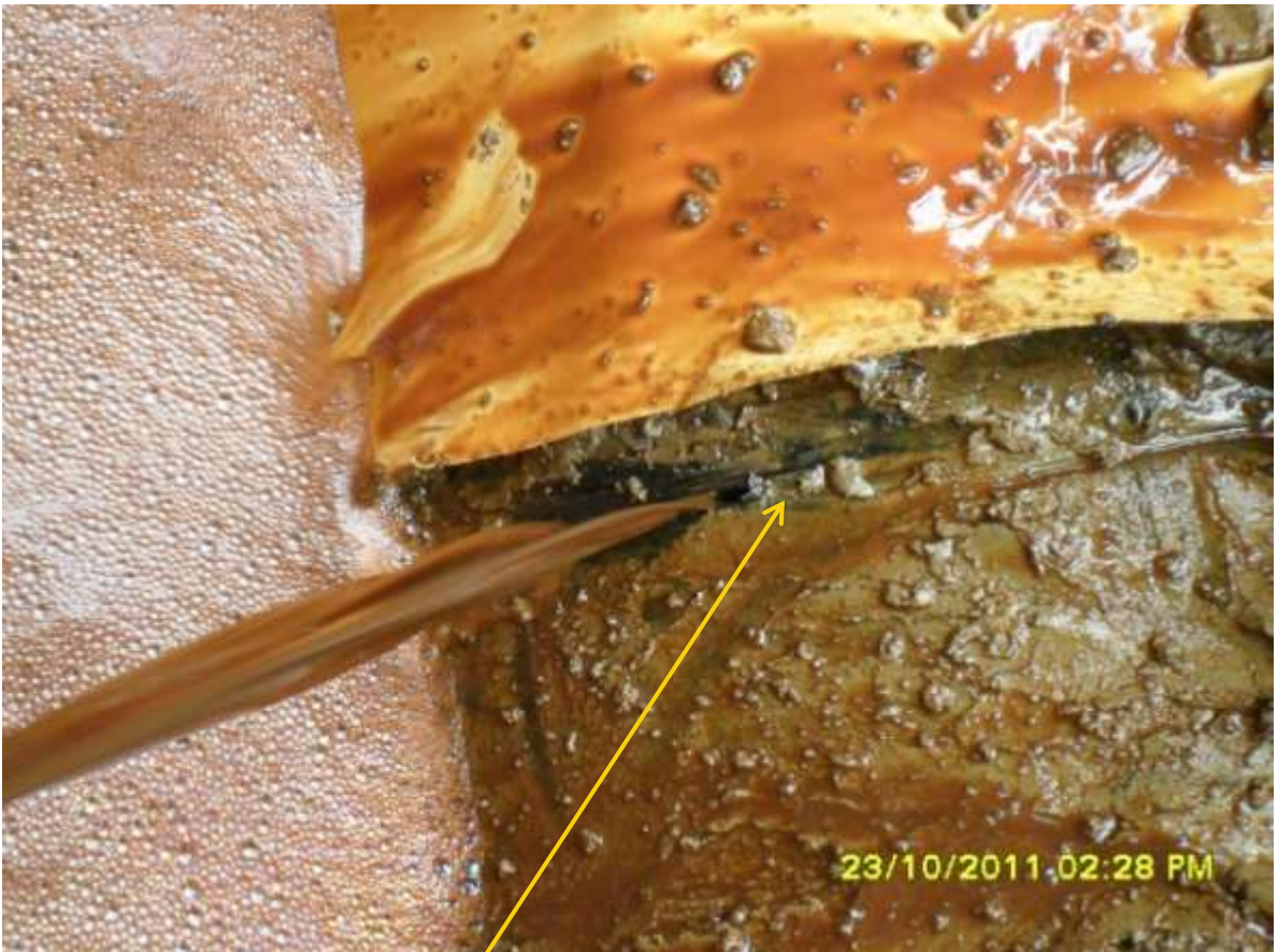
Close-up: Spill due to hacksaw cut on 14" Okordia-Rumuekpe pipeline at Ikarama. Picture was taken during Joint Investigation of 23 rd October, 2011.
