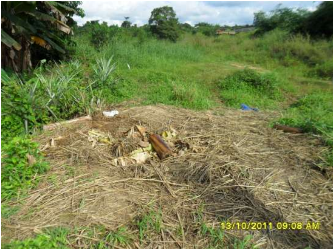
Overview: Location of suspected bunkering point on 12" Egbema-Oguta pipeline right of way at Eziosu. Picture taken during Joint Investigation of 13 th October, 2011.
