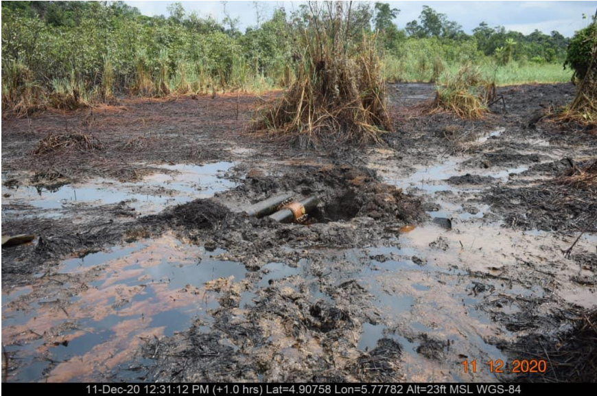
Overview: Part of spill impact on 6'' Seibuo Well 3 & 4 Bulkline at Agbidiana. Picture was taken during Joint Investigation on 11 th December 2020.
