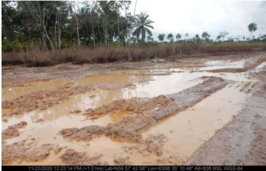
Overview: Part of spill impact on 20inch Kolocreek – Rumuekpe Trunkline at Owerewere. Picture was taken during Joint Investigation on 23rd November 2020.
