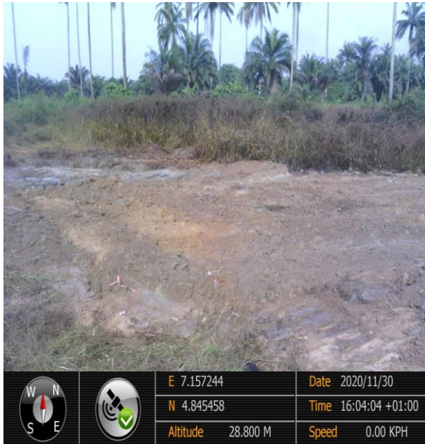
Overview: Part of spill impact on 12inch Imoriver 1 - Ogale Pipeline at Komkom. Picture was taken during Joint Investigation on 30th November 2020.
