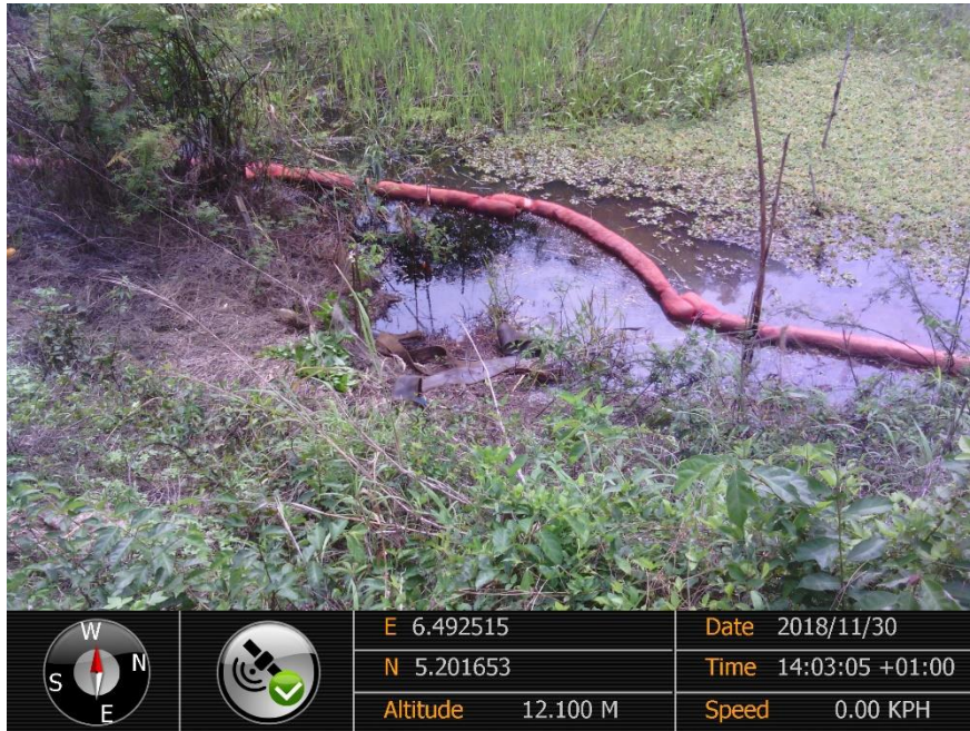
Overview: Part of spill impact on 4" Adibawa Well 12T Flowline at Edagberi. Picture was taken during Joint Investigation of 30 th November 2018.
