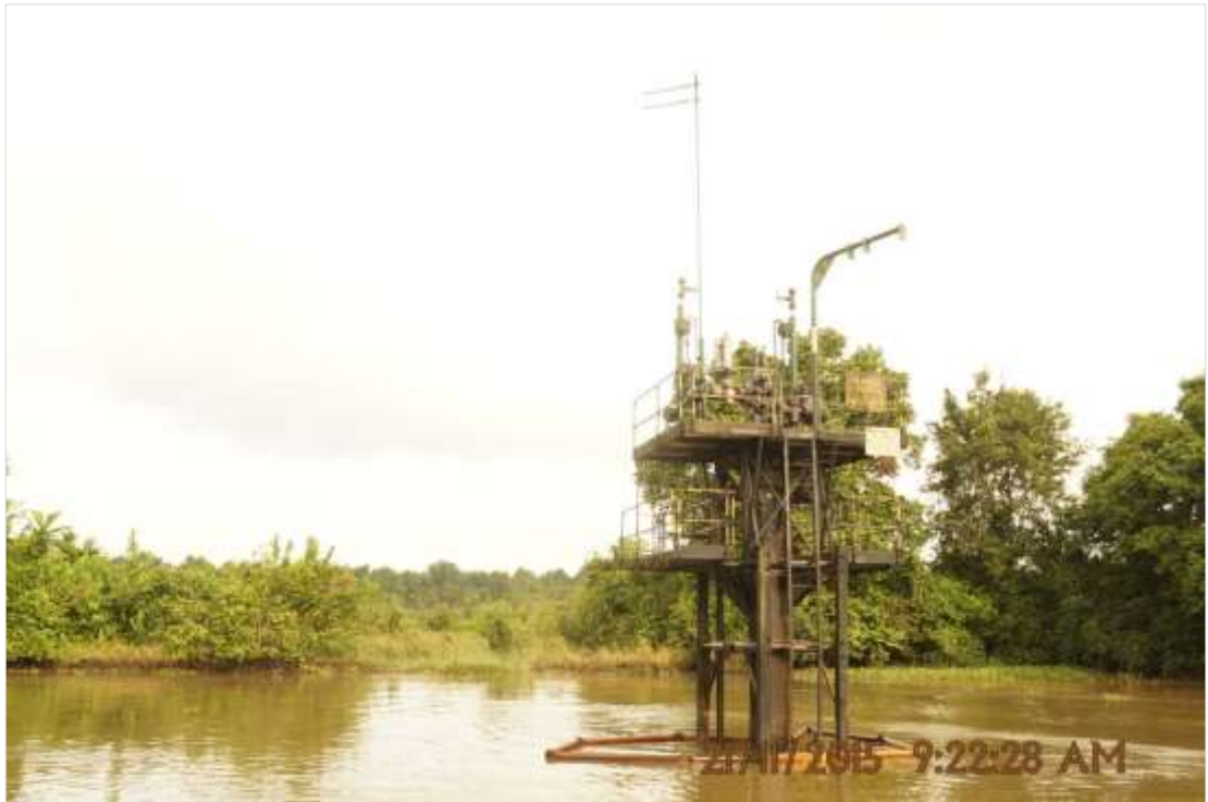
Overview: Location of spill on Tunu Kanbo Well4L Wellhead Right of Way at Agbidiana . Picture was taken during Joint Investigation of 21 st November 2015.
