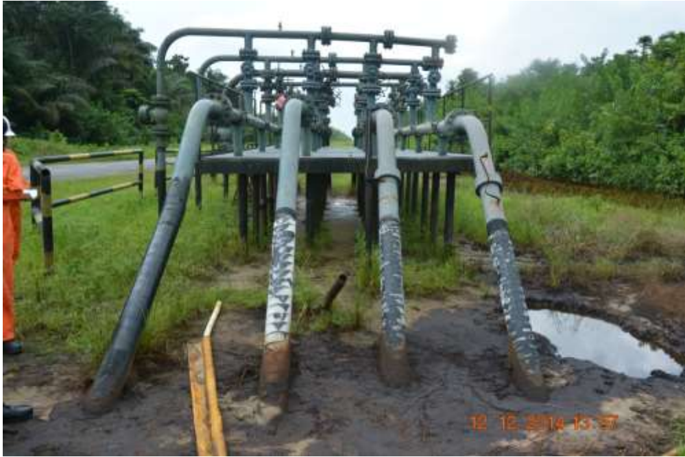
Overview: Part of spill impact on 6" Yokri Manifold7 Test Flowline Right of Way at Yokri. Picture was taken during Joint Investigation of 12 th of December 2014.
