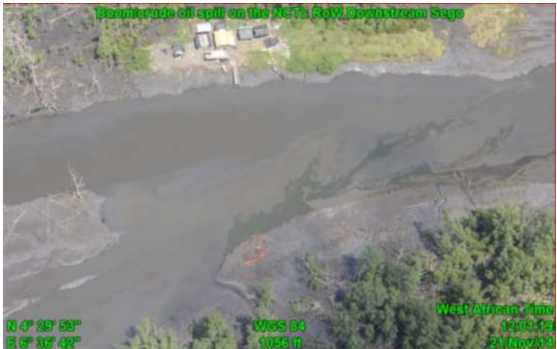
Overview: Part of spill impact on 24" Tora - Segoo Pipeline Right of Way at Segoo. Picture was taken during Overfly of 21 st November 2014.
