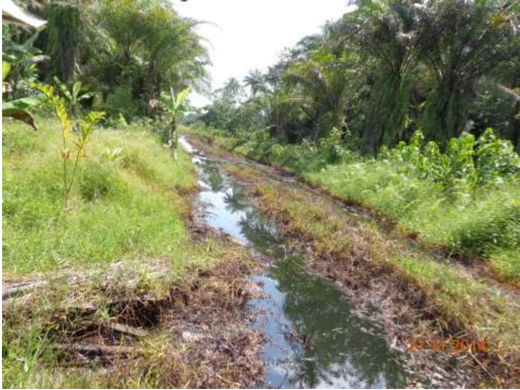
Overview: Part of spill impact on 14" Okordia-Rumuekpe Pipeline Right of Way at Ikarama. Picture was taken during Joint Investigation of 21 st November 2014.
