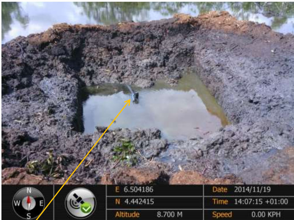
Close-up: Illegal fitting on 6" Odeama-Tora Pipeline at Bassambiri. Picture was taken during Joint Investigation of 19 th November 2014.
