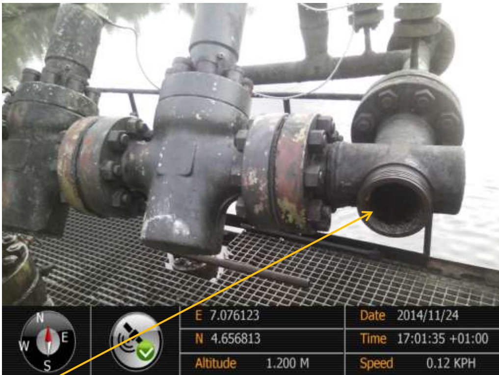
Close-up: Position of missing bean cap on Alakiri Well19T Wellhead at Ofiomina-Ama. Picture was taken during Joint Investigation of 24 th November 2014.
