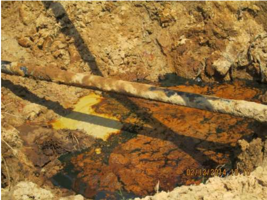
Overview: Part of spill impact on 4" Etelebou Well 11T Flowline Right of Way at Ogboloma. Picture was taken during Joint Investigation of 2 nd December 2014.
