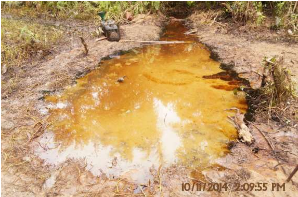
Overview: Part of spill impact on 20" Otumara – Escravos Pipeline Right of Way at Ogidigben. Picture was taken during Joint Investigation of 10 th November 2014.
