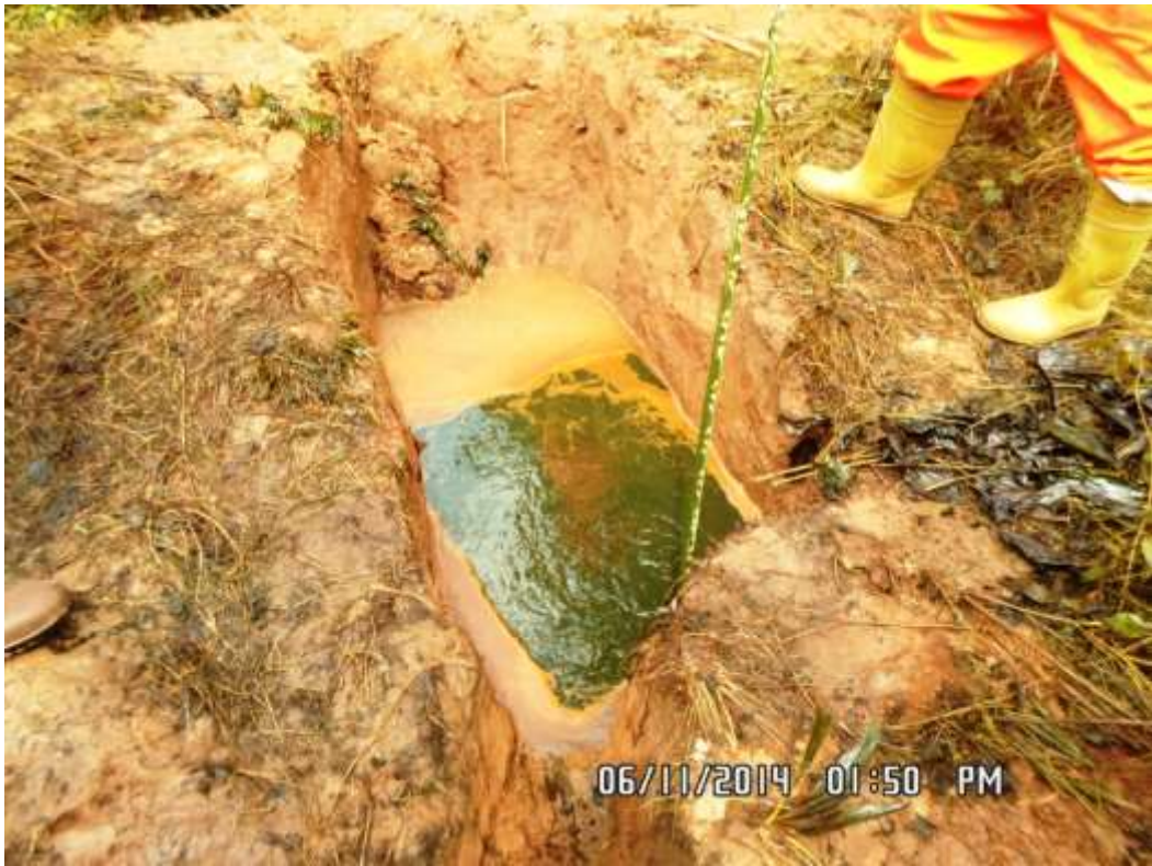
Overview: Spill impact on 28" Nkpoku-Bomu Pipeline Right of Way at Norkpo. Picture was taken during Joint Investigation of 6 th November 2014.
