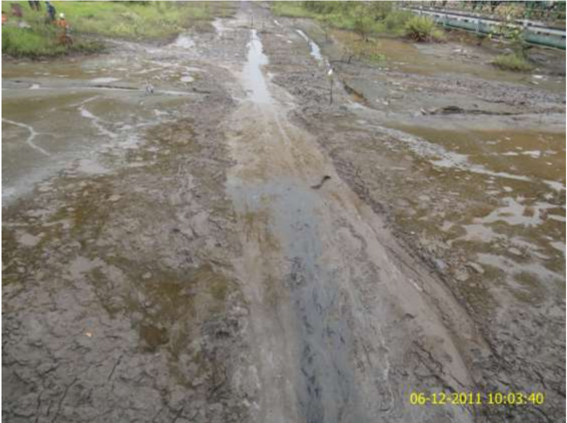
Overview: Part of spill impact on Awoba Well8T flowline at Bille. Picture was taken during Joint Investigation of 6 th December, 2011.
