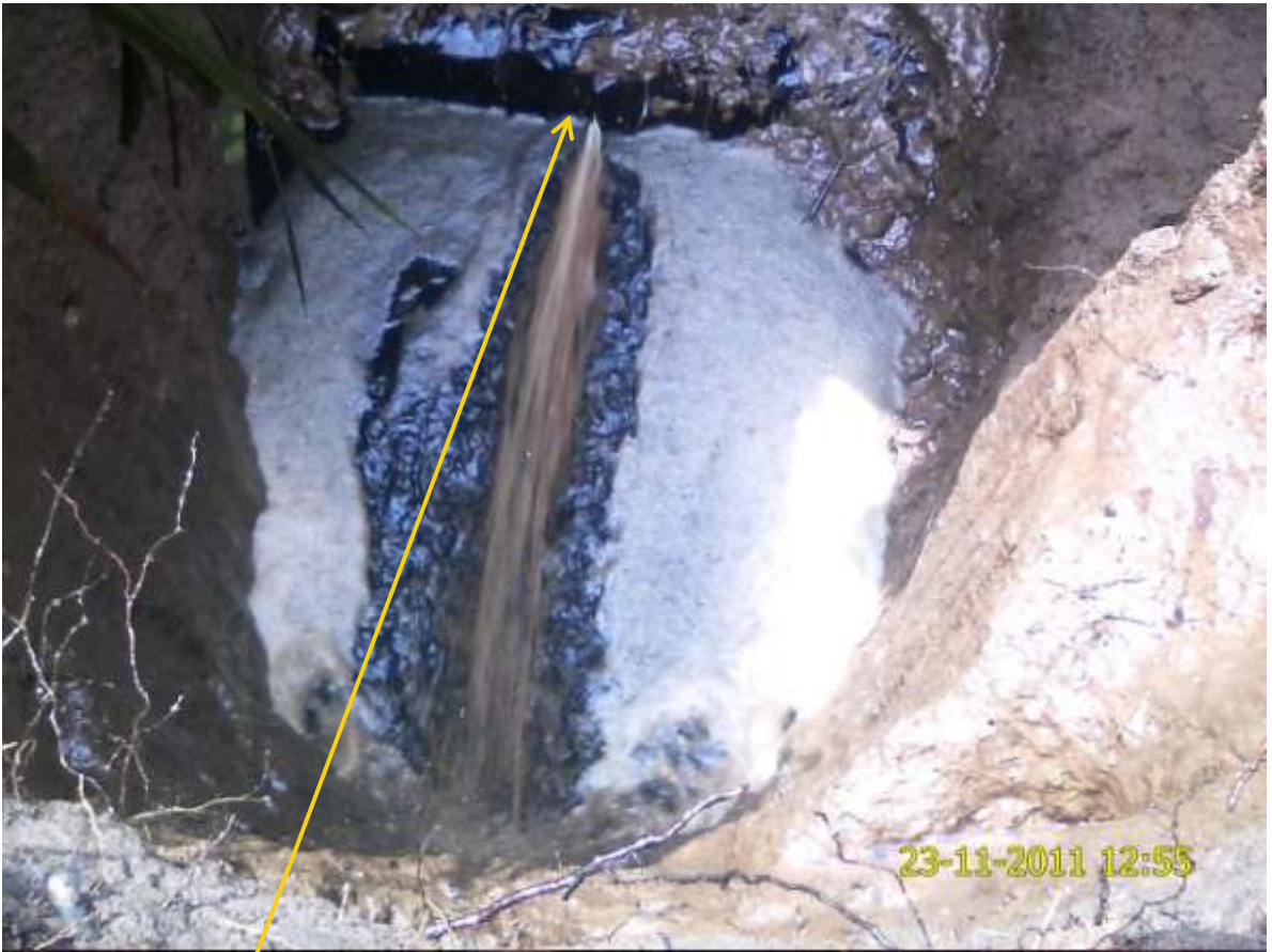
Close-up: Spill due to hacksaw cut on 6" ObigoNorth-Ogale pipeline at Ogale. Picture was taken during Joint Investigation of 23 rd November, 2011.
