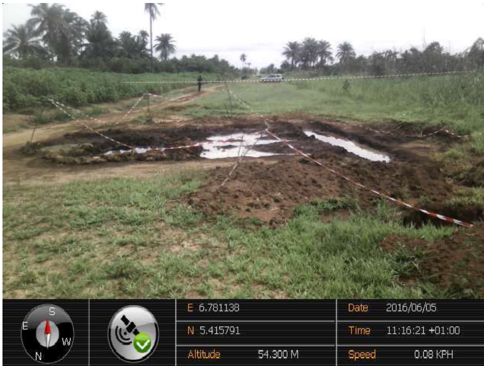
Overview: Part of Spill Impact on 16" Egbema-Assa Pipeline Right of Way at Ekpeagah. Picture was taken during Joint Investigation of 5 th June 2016.
