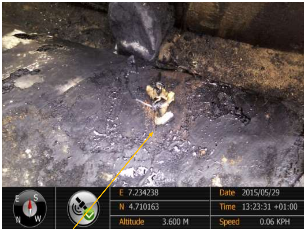
Close-up: Hacksaw cut on 28" Nkpoku-Bomu Pipeline at Kpoghor. Picture was taken during Joint Investigation of 29 th May 2015.
