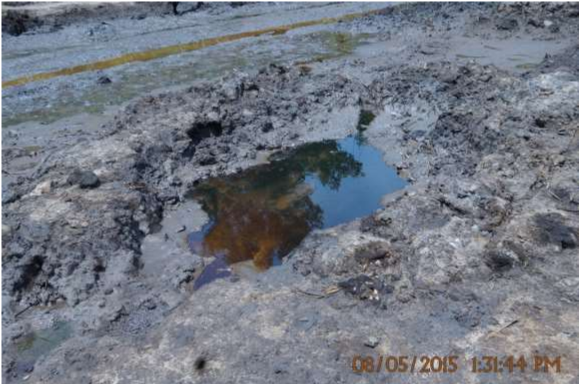
Overview: Part of spill impact on 20" Otumara-Escravos Pipeline Right of Way at Ugboegungun. Picture was taken during Joint Investigation of 8 th May 2015.
