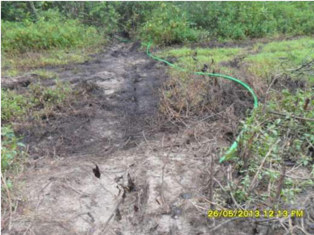
Overview: Part of spill impact on 24" Nkpoku-Bomu pipeline right of way at Egbalor. Picture was taken during Joint Investigation of 26 th May 2013.
