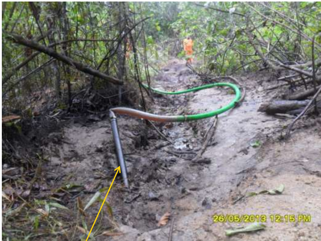
Overview: Part of spill impact on 24" Nkpoku-Bomu pipeline right of way at Egbalor. Illegal hoses can be seen connected to illegal bunkering point.
