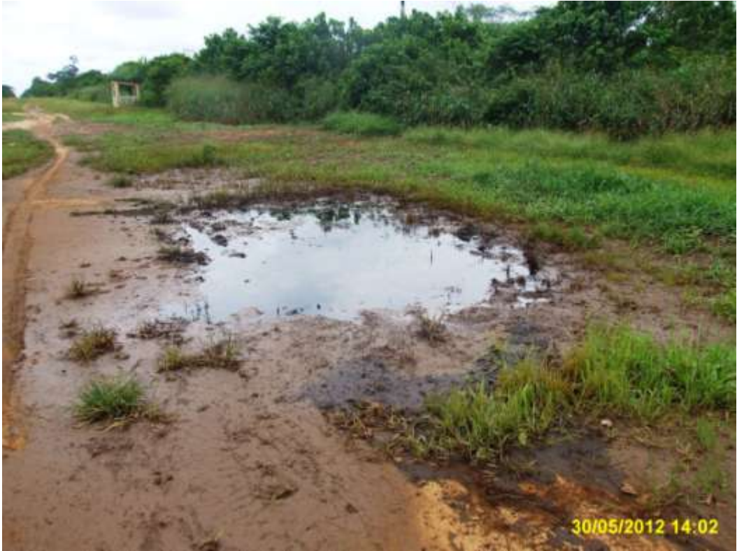
Overview: Part of spill impact on 18" Assa-Rumuekpe pipeline right of way at Egbeda. Picture was taken during Joint Investigation of 30 th May 2012.
