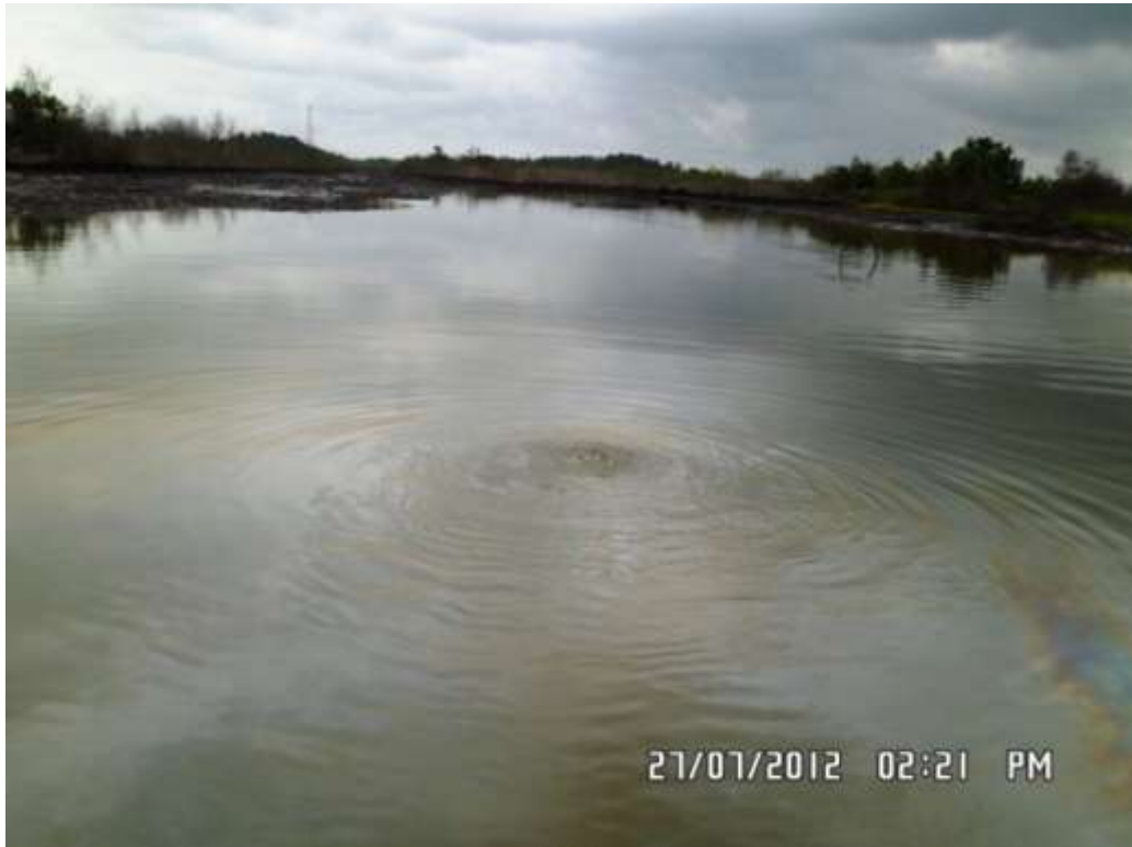
Overview: Part of spill impact on 8" Cawthorne Channel 2 delivery line right of way at Tigerkiri. Picture was taken during Joint Investigation of 27 th July 2012.
