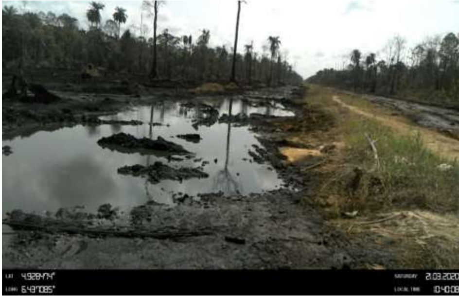
Overview: Part of spill impact on Old 20" Kolocreek – Rumuekpe Pipeline at Odau-KP9. Picture was taken during Joint Investigation of 21 st March 2020.
