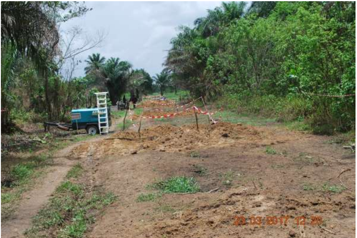
Overview: Part of spill impact on 4" Obele-Ibaa Pipeline Right of Way at Ibaa. Picture was taken during Joint Investigation of 23 rd March 2017.
