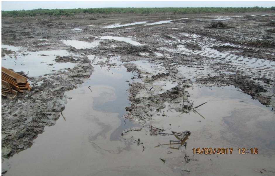
Overview: Part of spill impact 28" Bomu-Bonny Trans Niger Pipeline at Owokiri. Picture was taken during Joint Investigation of 19 th March 2017
