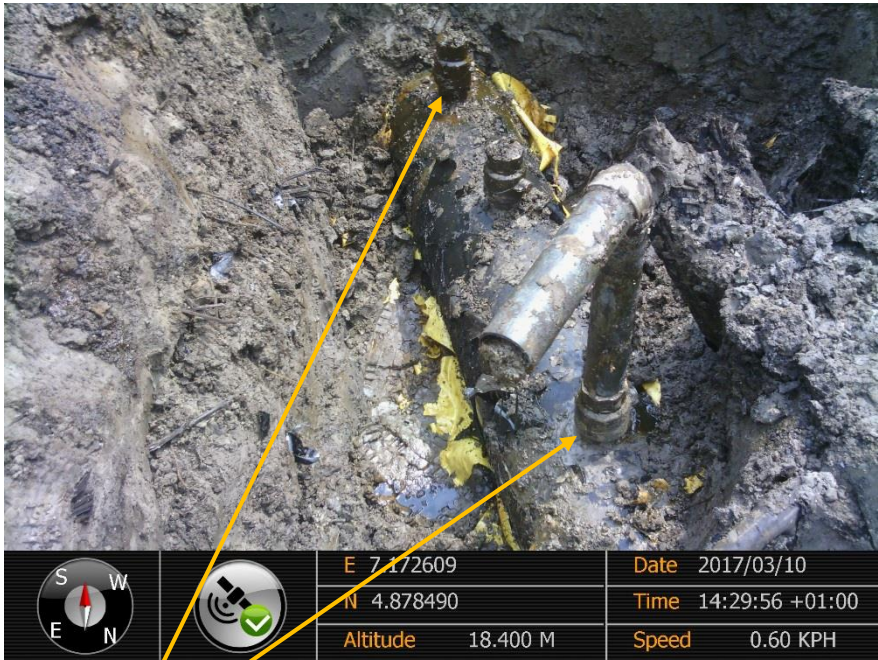
Close-up: Leaking Illegal fittings on 12" Imo River-Ogale Pipeline at Komkom. Picture was taken during Joint Investigation of 10 th March 2017.
