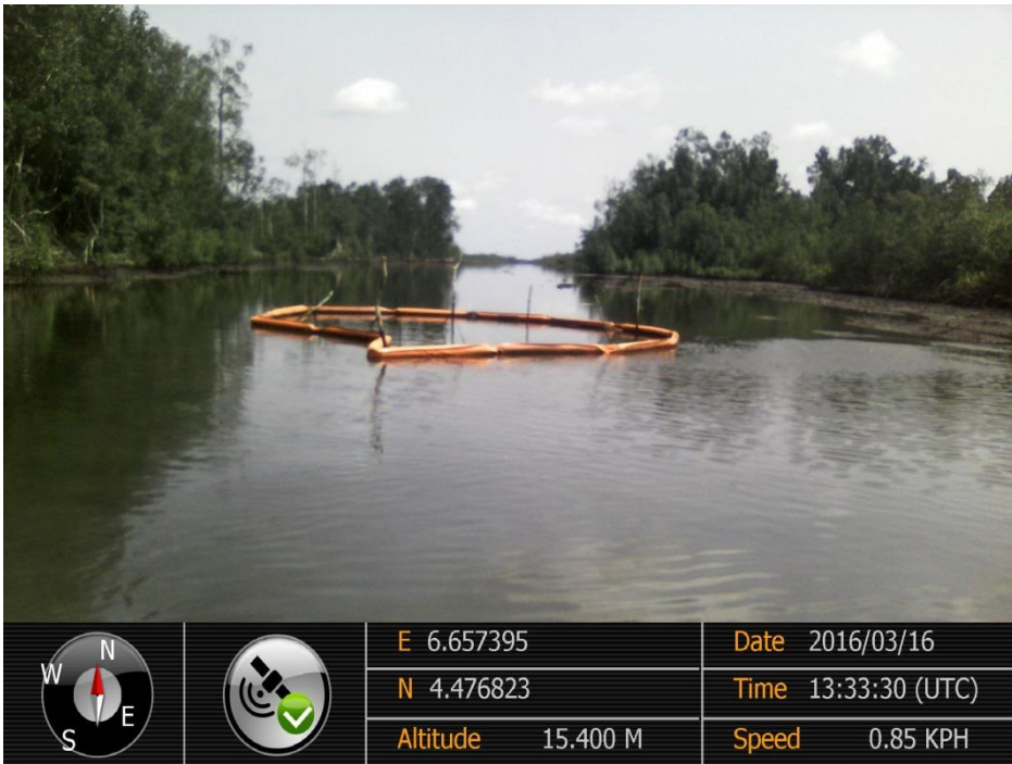
Overview: Part of spill impact on 8"Belema-Sego Delivery line at Offoinama. Picture was taken during Joint Investigation of 16 th March 2016.
