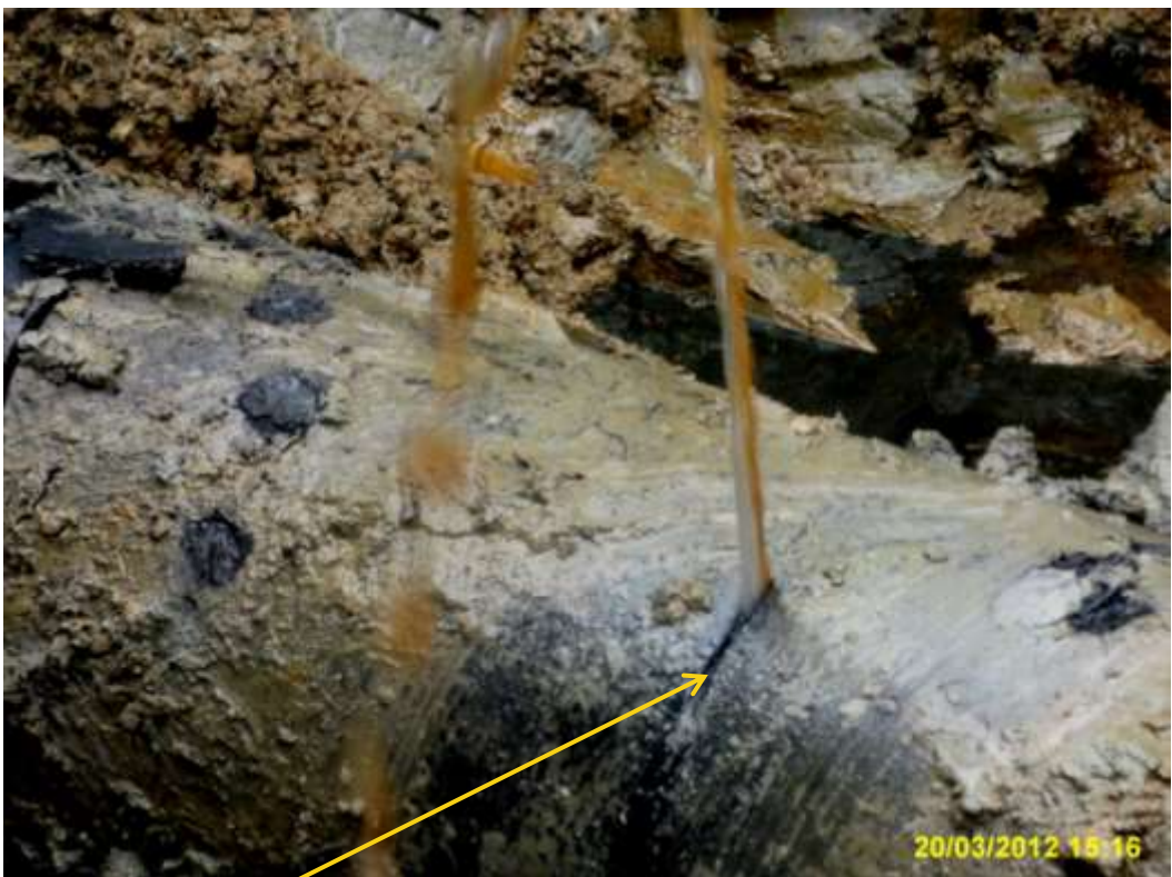
Close up: Hacksaw cut on 16" Nun River - KoloCreek pipeline at Oporoma. Picture was taken during Joint Investigation of 20 th March 2012.
