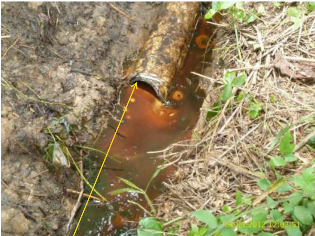
Close up: Cut section on Ubie Well9S flowline at Idu-Ekpeye. Picture was taken during Joint Investigation of 4 th April 2012.
