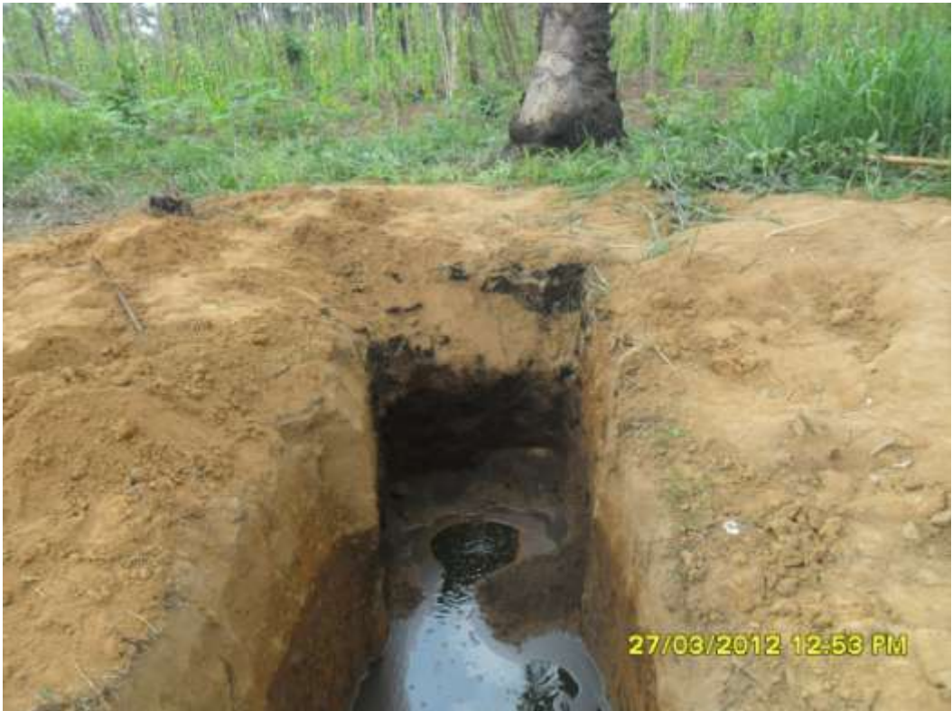
Overview: Part of spill impact on 24" Nkpoku-Bomu pipeline right of way at Bera. Picture was taken during Joint Investigation of 27 th March 2012.
