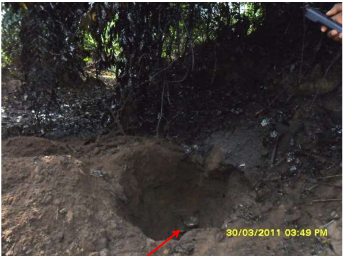
Close-up: Picture showing illegally welded point on 6" Well 59T flow line at Imo River. Picture taken during Joint Investigation of 30 th March, 2011.
