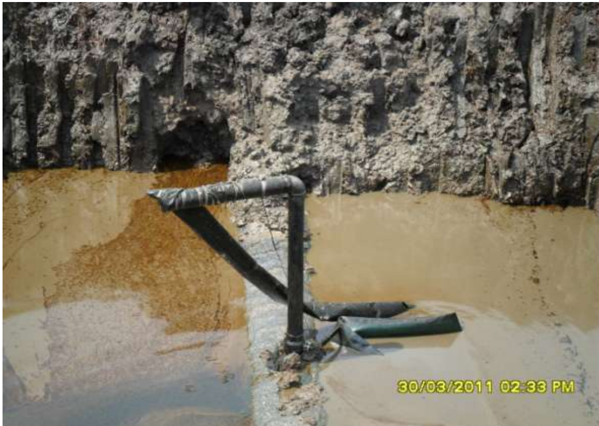
Overview: Extent of the spill incident impact on 24in Bomu-Bonny pipeline at Bodowest. Spill site showing oil theft hose still attached to illegal off take point.
