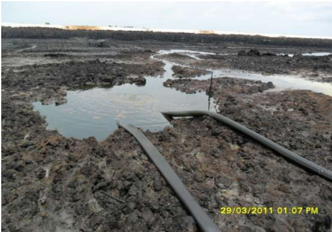
Overview: Extent of the spill incident impact on 28in Bomu-Bonny pipeline at Bodowest. Spill site showing oil theft hoses still attached to illegal off take points.
