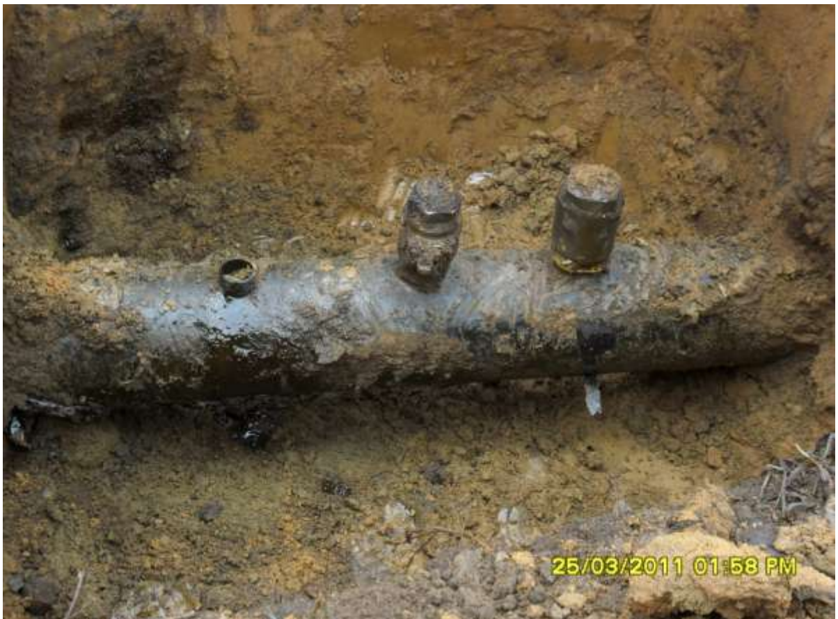
Close-up: Spill was due to illegally welded point on 8" Obigbo-North Pipeline at Obigbo. Picture taken during Joint Investigation of 25 th March, 2011.
