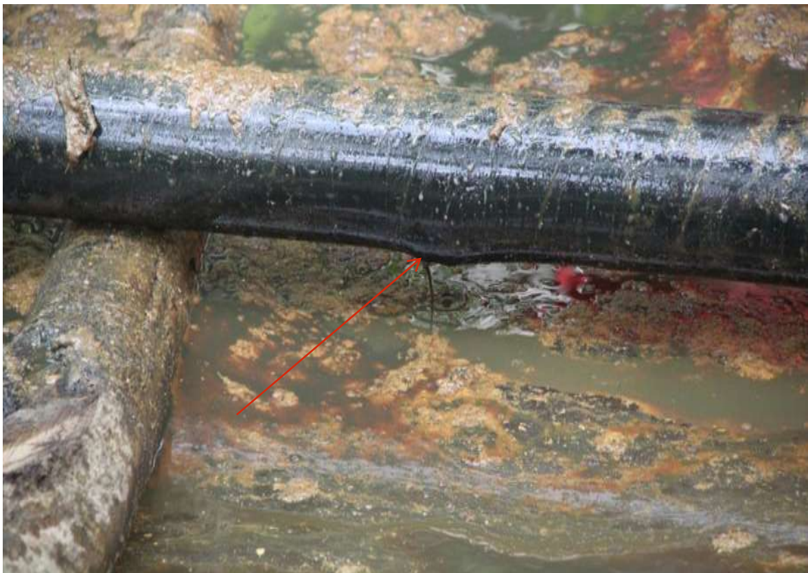
Close-up: Spill due to corrosion on Opukushi W-34T flowline ROW.. Picture taken during Joint Investigation of 18 th March, 2011.
