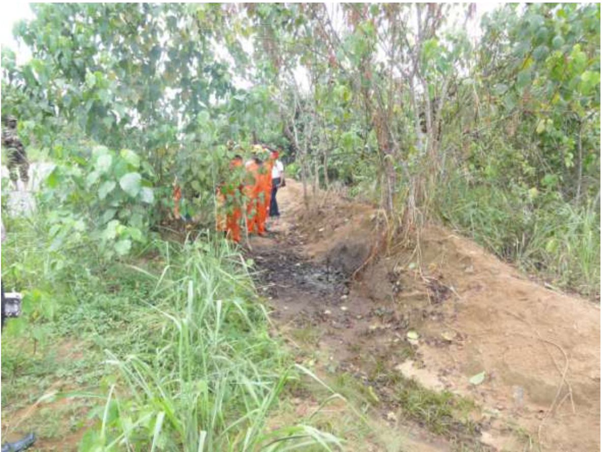
Overview: Extent of the spill incident impact at Imo River 1 Well 59T flowline right of way. Picture was taken during JIV of 15 March 2011
