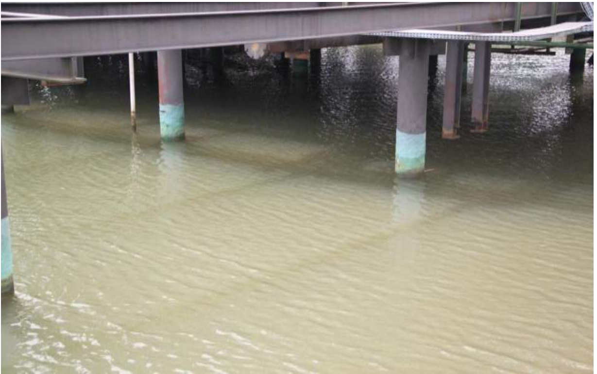
Overview: Showing spill point environment at Batan Flowstation in Batan. Picture was taken during JIV of 11 March 2011
