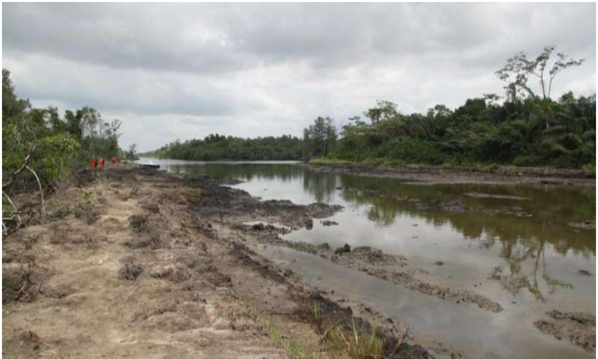
Overview: Extent of the spill incident impact at 28" Trans Forcados Pipeline route in Chanomi. Picture was taken during JIV of 10 March 2011
