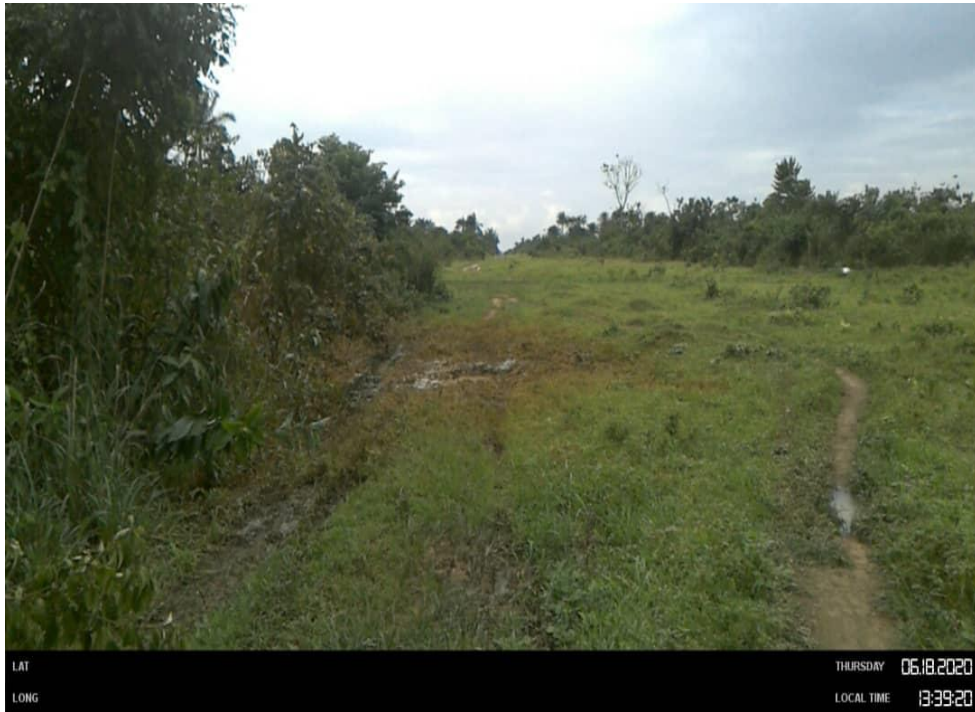
Overview: Part of spill impact on 8" Nkali - ImoRiver Deliveryline at Odagwa. Picture was taken during Joint Investigation 18th June 2020.
