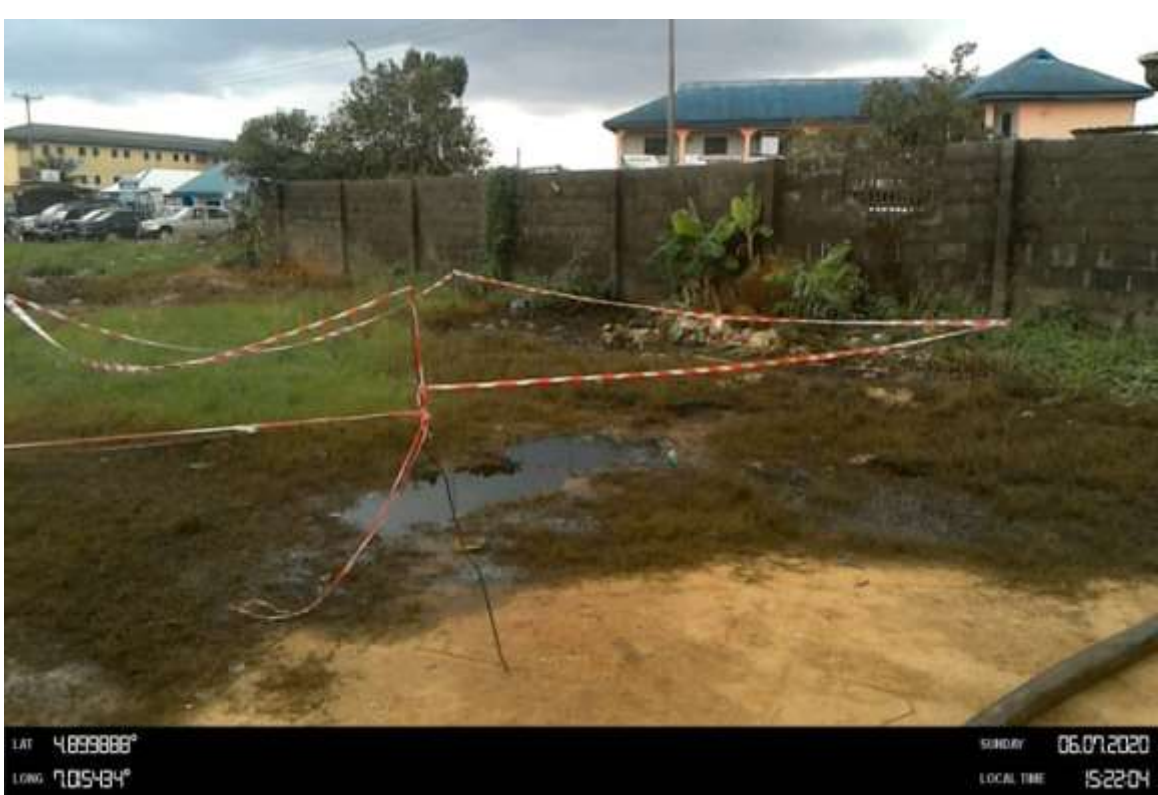
Overview: Part of spill impact on 28" Nkpoku Bomu Pipeline at Rumuowha. Picture was taken during Joint Investigation 7th June 2020.
