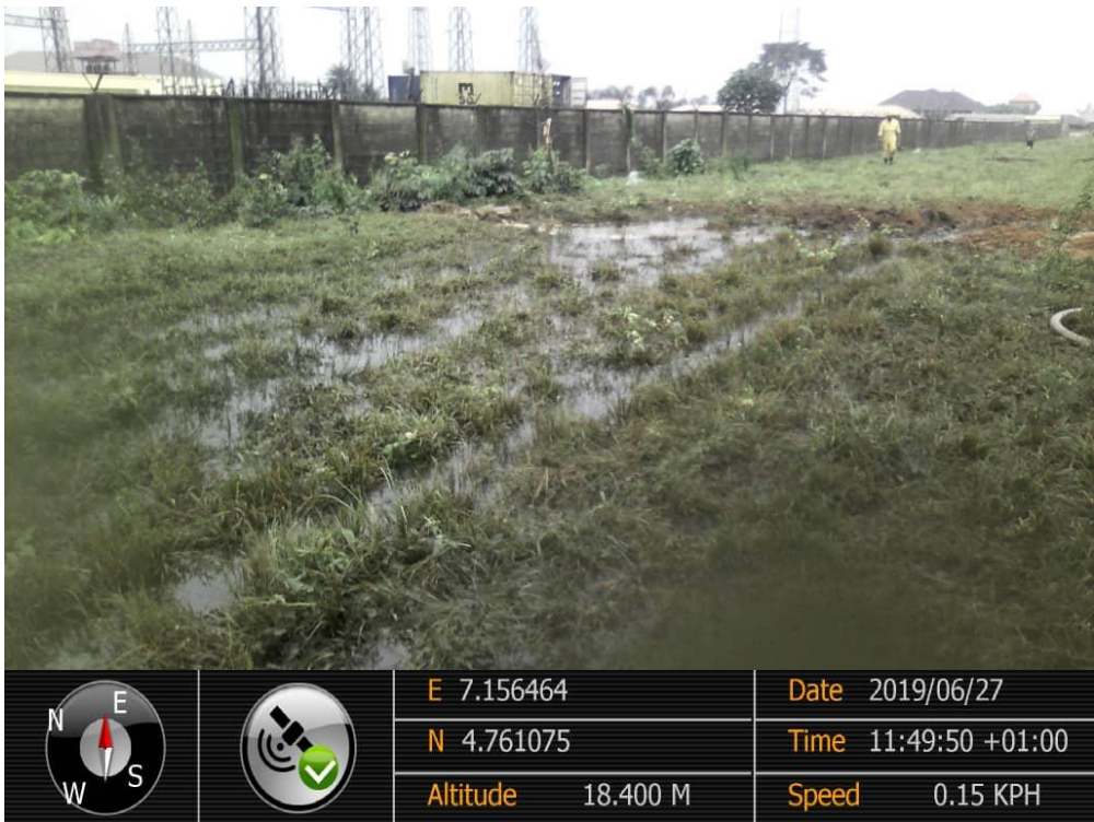
Overview: Part of spill impact on 28'' Nkpoku - Bomu Pipeline Right of Way at Ejamah – Ebubu. Picture was taken during Joint Investigation of 27 th June 2019.
